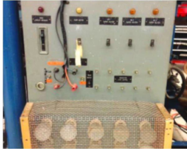
Figure 7: Generator and Load
